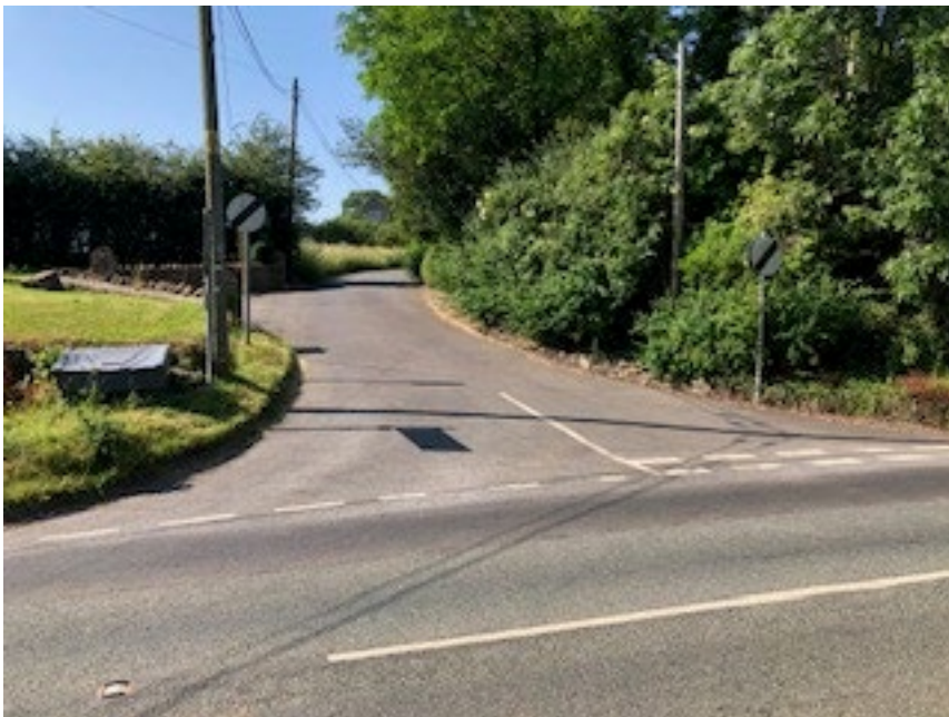
Fig 4. A366/TR junction – driveway immediately on L then narrows
